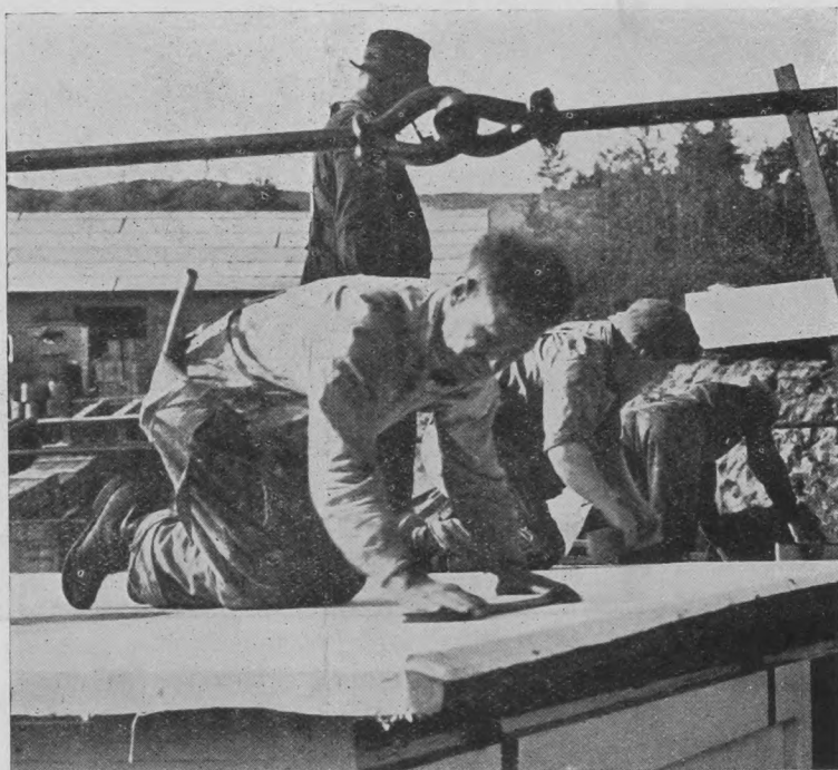
Putting the finishing touches on the pilot house.
